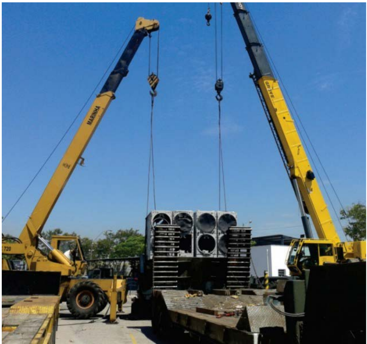
Photo 8 - Joint operation of two cranes on wheels of the BNRJ to remove the missile launcher (20t) ASROC from above the CavMec of the CFN
