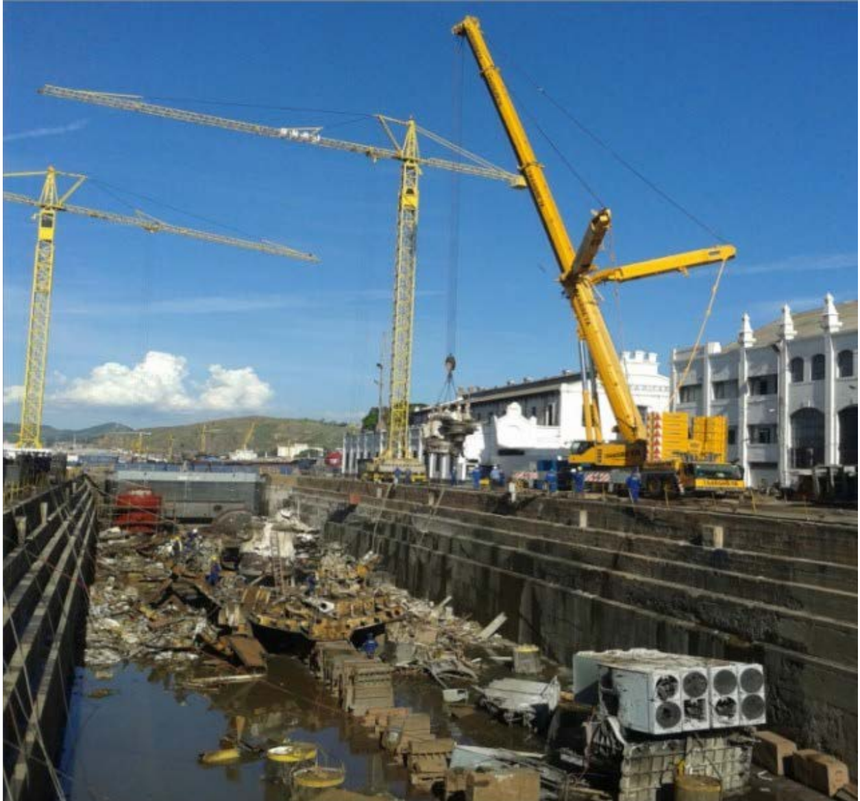
Photo 7 - Large capacity (up to 440t) contracted crane removing one of the boilers
